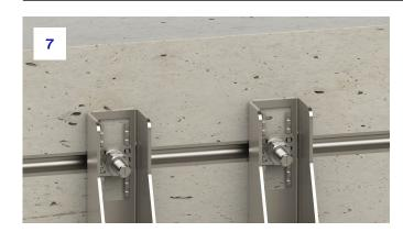
**4.** Nuts and form B washers can then be loosely placed onto the bolts and the level adjusted as required. The alpha washer can be spun 180° to allow for fine adjustment if required. The nut can then be tightened to the correct torque setting of 25Nm.
