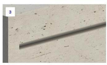
**3.** No filler or concrete should be left within the channel. Any remaining concrete should be scraped out. It is important that no power tools are used for this and sufficient care is taken of the concrete in the surrounding area.
