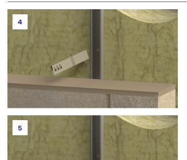
4. Rotate ACS 4000 range tie into channel lips.
