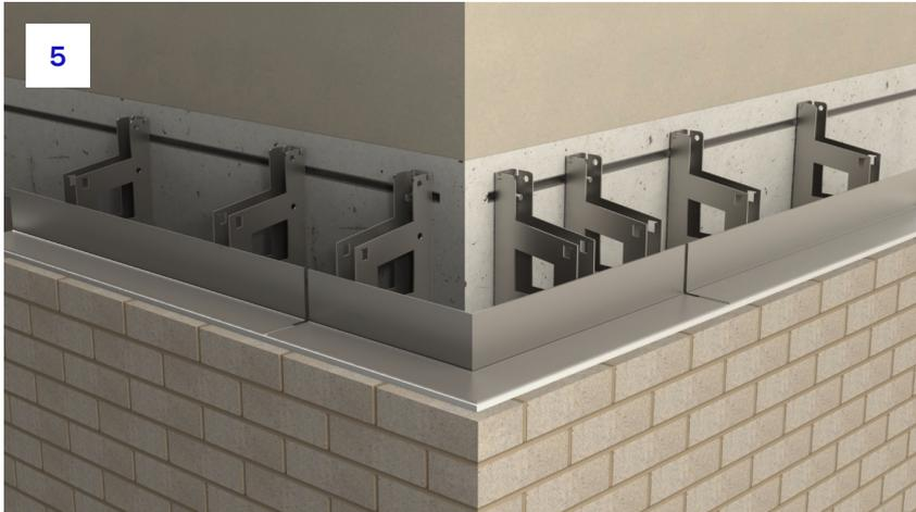
5. Continue to install further pieces of Intex™ brackets and angle following ACS approval drawings, allowing for around a 10mm gap between units. Each angle should be levelled to the value shown upon the ACS drawings. A string line is commonly used to assist with installation.
