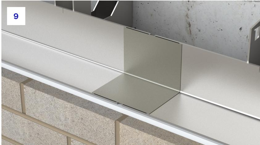
**9.** The Intex™ jointing piece should be pushed down into the tape to ensure good adhesion and to prevent water from being able to pass through.
