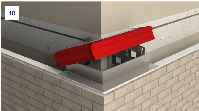
10. The tray should be rotated around to allow the formed section to be inserted into the bracket notches. The tray can be temporarily slid to the left to allow for easy rotation.
