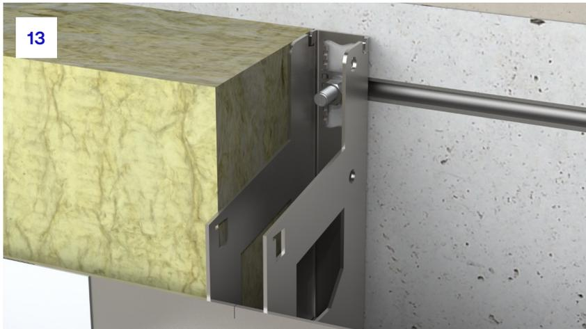
**13.** Thermal insulation should be installed tight up to the edge of each bracket and secured back to the structure following the manufacturer's instructions. Maximum gaps to the Intex™ barrier should be adhered to.
